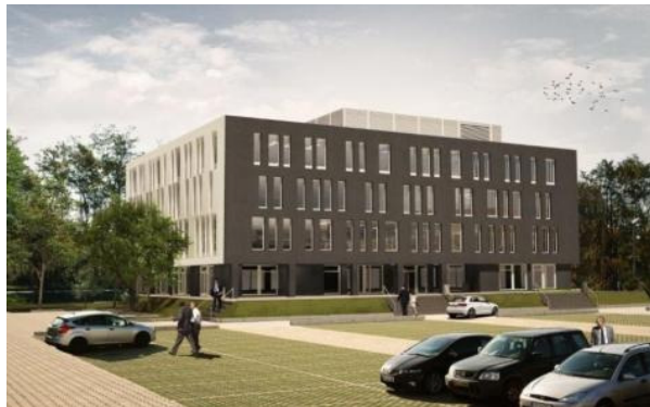
Nickel Technology Park Poznań , plans to open the new Business Services Centre in May 2015. Image: NTPP
