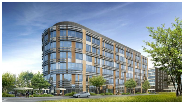
West Point 120 will welcome first tenants in 2016. Image: Bouygues Immobilier Polska
